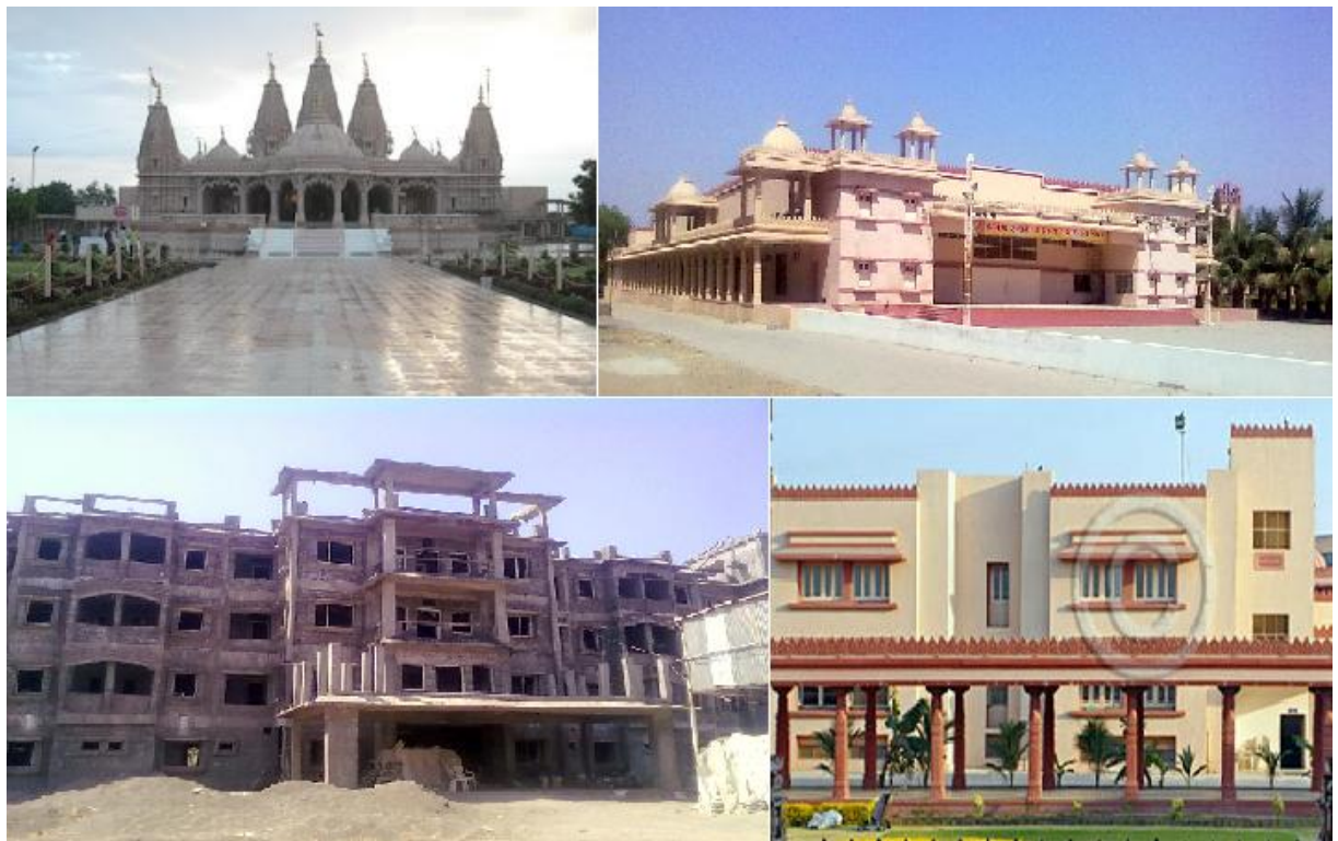
Fig. 8 Structures in which fly ash bricks are used
